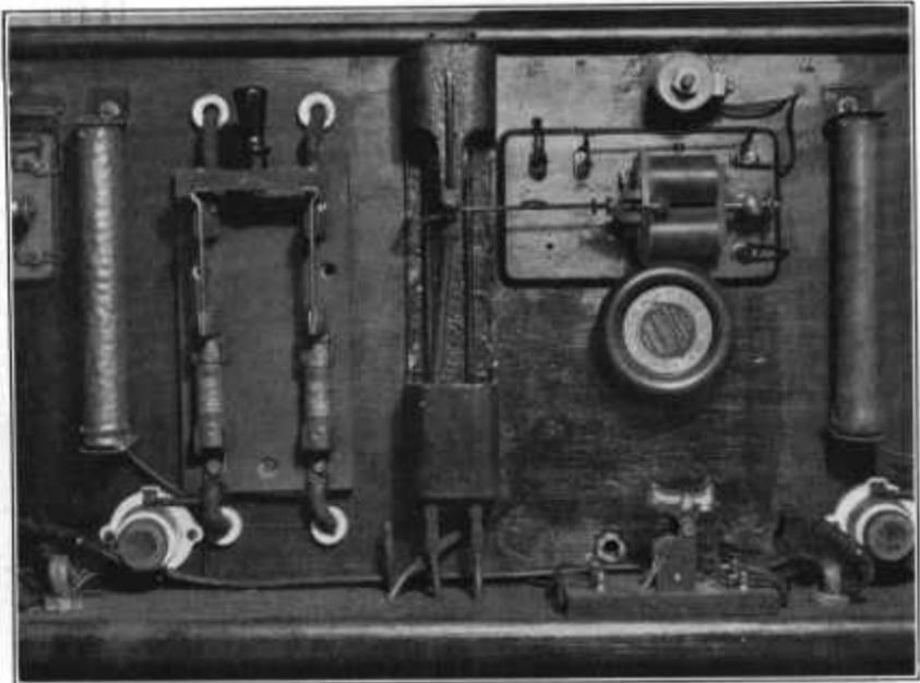
FIGURE 3.—Rocking funnel and relay as they appear on switchboard above light case. The rectifier unit, here functioning as a check valve, is just above the relay
