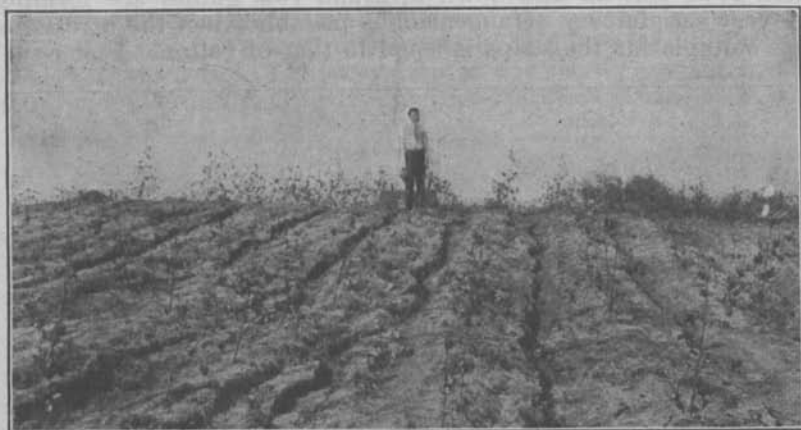
FIGURE 5.—Land unprotected from erosion, showing row gullies forming
