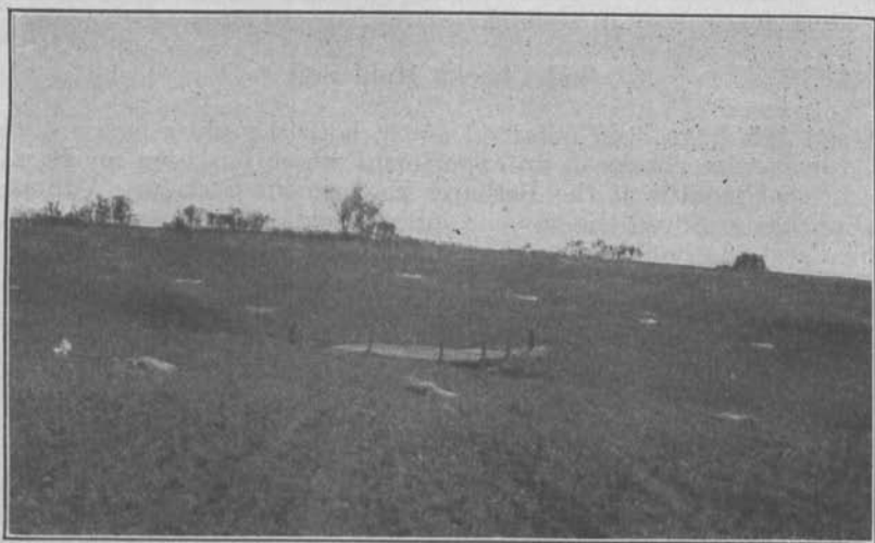
FIGURE 3.—Woven-wire dam in foreground with sod barriers in background at Bethany Soil Erosion Experiment Station. A considerable quantity of soil has been deposited above each sod check and also above the woven-wire dam
