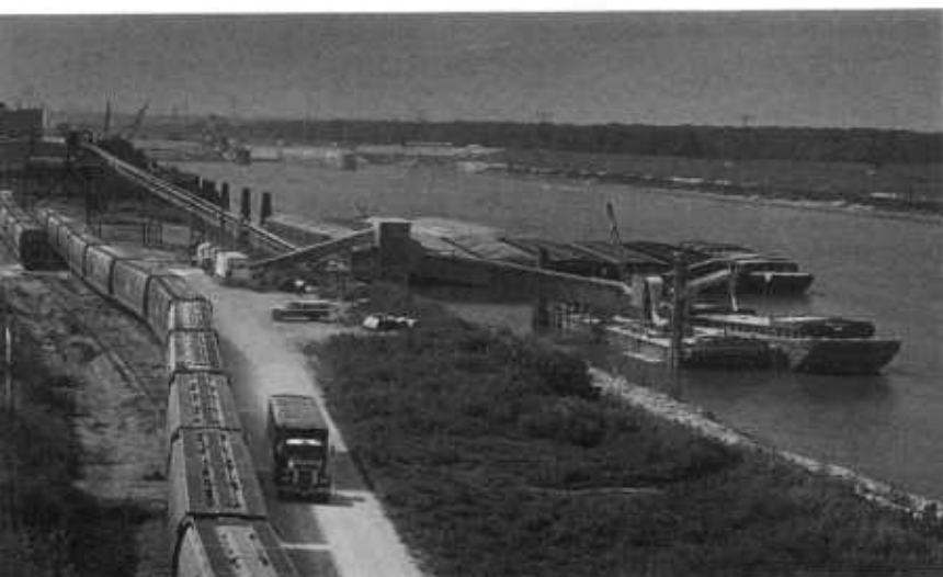
Unit trains, like the one at the left, usually consist of 25 or more jumbo-covered hopper cars. They are capable of moving large quantities of grains to terminal facilities such as this one where barges are being loaded. Most agricultural commodities transported by rail for export move in unit trains.
