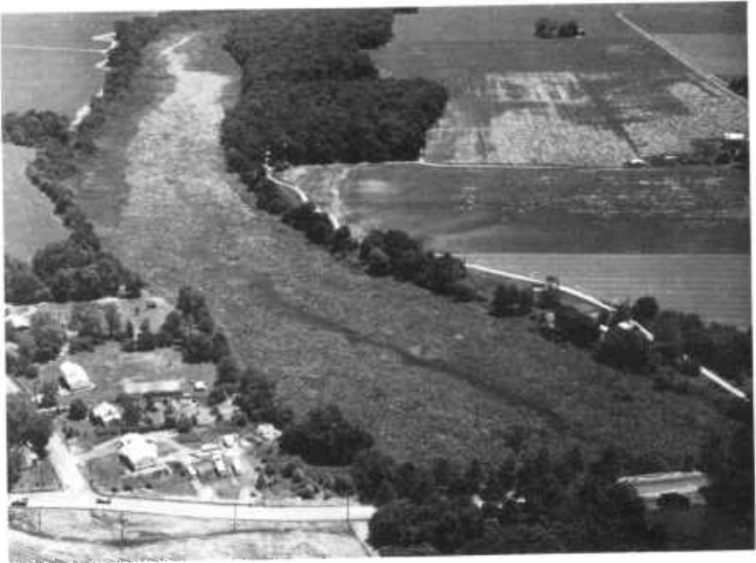
This New Jersey coastal plain pond suffered from heavy water-weed growth due to siltation and excessive runoff containing fertilizers. Various governmental agencies combined efforts to improve drainage of the 600 by 1,500 foot pond. (Clarence Deland, SCS, NJ-40,498)
