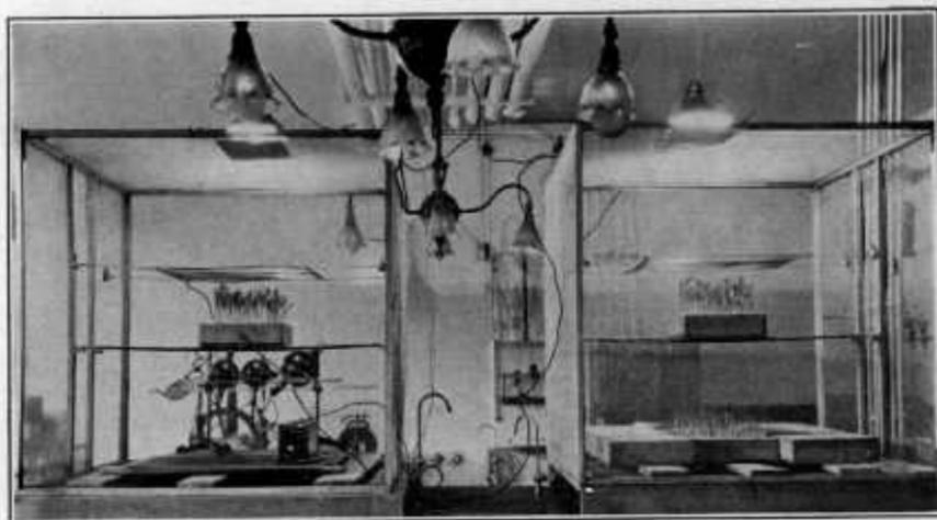
FIGURE 1.—Apparatus used in electric treatment of growing plants in 1924 and 1925. One side of each cage has been removed to expose the interior arrangements
