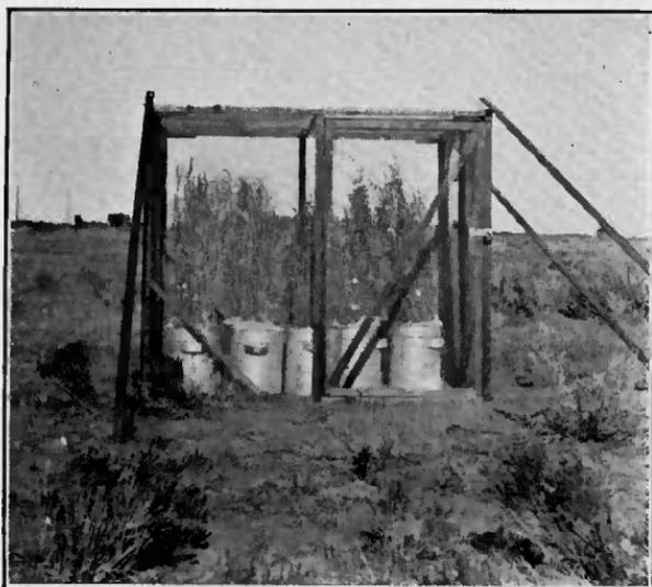
FIGURE 7.—Apparatus used in subjecting inoculated wheat and barley flowers to the low humidity of the desert
