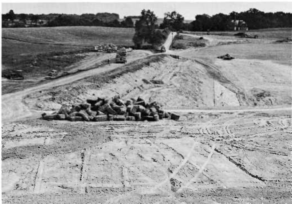
Engineers of the Soil Conservation Service checked the contractors' work on the dams, nine of which were planned for the watershed, at a cost of about 900 thousand dollars. The surfaces of the completed dams are protected by seeding with grass to prevent erosion. Baled hay is spread as a mulch to help the grass get started.
