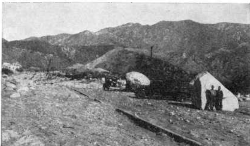
FIGURE 33.—Boulders weighing 60 tons each deposited on a street of La Crescenta by the New Year's flood from Dunsmere Canyon.
