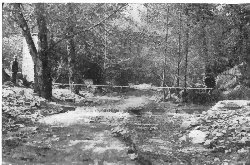
FIGURE 35.—Arroyo Seco Creek, undamaged by storm run-off from forest-covered watershed adjacent to the burned area. White line shows high-water mark of the New Year's storm. The water, being clear and controlled, was harmless. Compare with figure 34.
