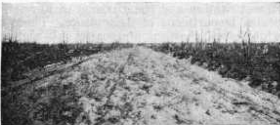
FIGURE 48.—Newly constructed protection road widened for fire control.
