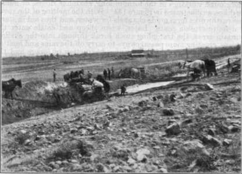
FIGURE 156.—Expensive break in irrigation ditch near Kennewick, Wash., caused by water finding its way through burrows made by pocket goppers
