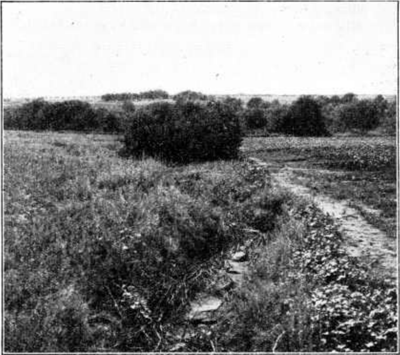
FIGURE 76.—Showing silt deposited to top of brush in gully shown in Figure 75
