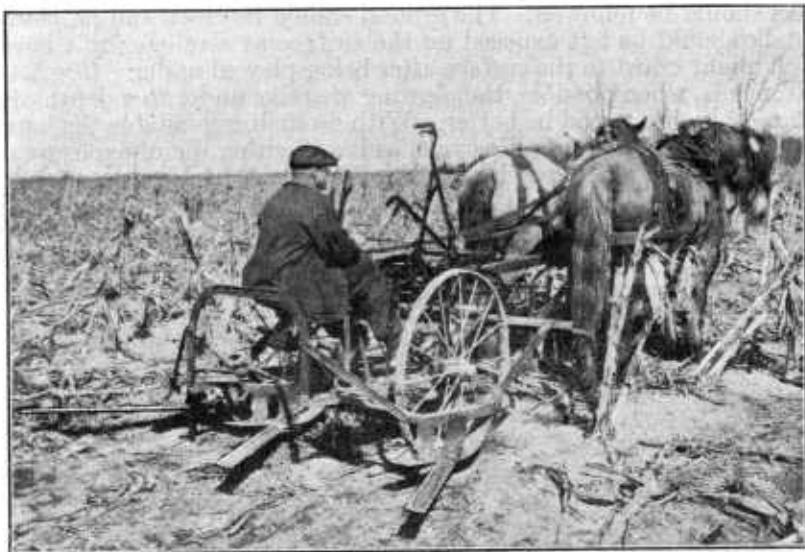
FIGURE 25.—A wheel-type stalk shaver cutting three rows at a time
