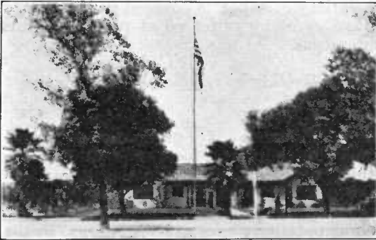
FIGURE 147.—Administration building of the United States Rabbit Experiment Station operated by the Bureau of Biological Survey at Fontana, Calif., to determine the best methods of producing rabbits for food and fur. The structure is of white stucco with a red tile roof
