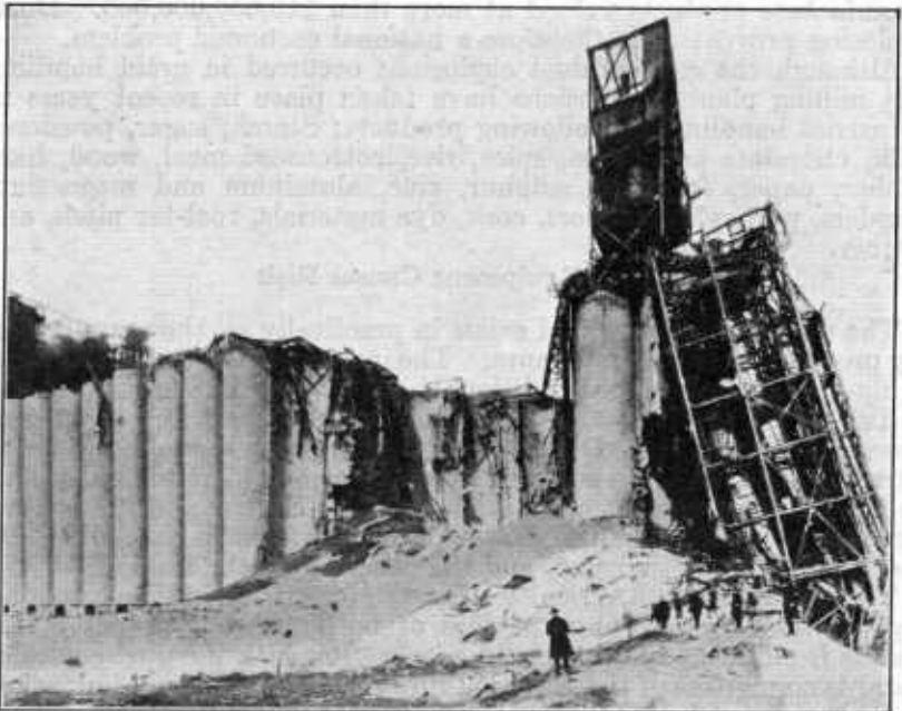
FIGURE 75.—The world's largest grain elevator, 10,000,000 bushels capacity, located at South Chicago, Ill., wrecked by a grain-dust explosion. The explosion killed six men and resulted in $4,500,000 property damage
