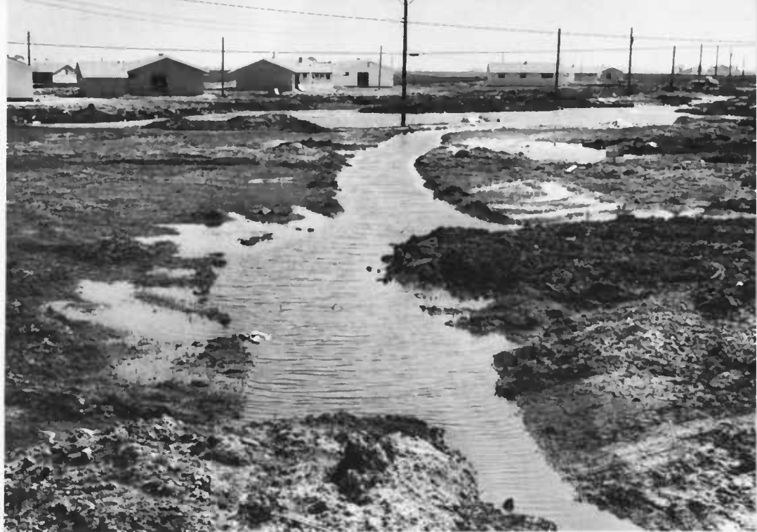
Poor drainage is manifest in this subdivision in Cook County in Illinois.
