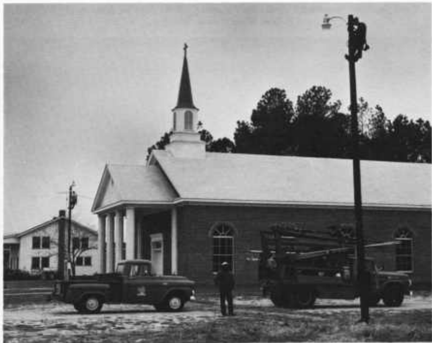
A church near Lake City, S.C., receives free yard light from the Santee Electric Cooperative.
