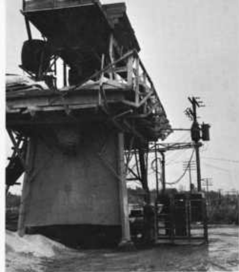
A concrete-block plant on Santee's lines is typical of small rural industries that are springing up in the electrified countryside.
