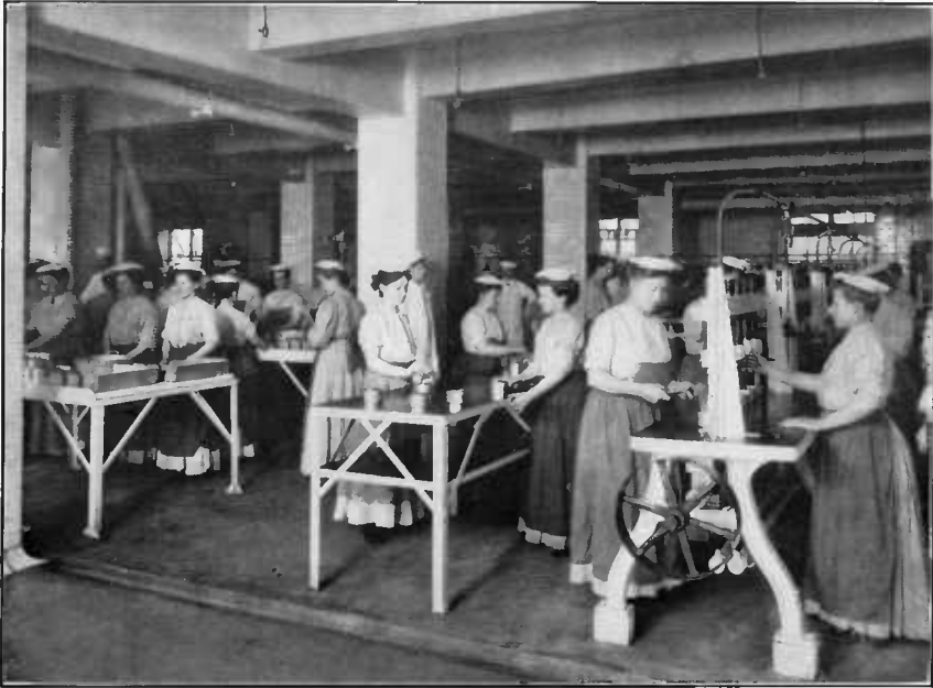
FIG. 1.—CAPPING THE CANS.
