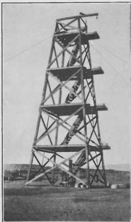
FIG. 1.—Tower No. 1, 1,500 FEET INLAND.
