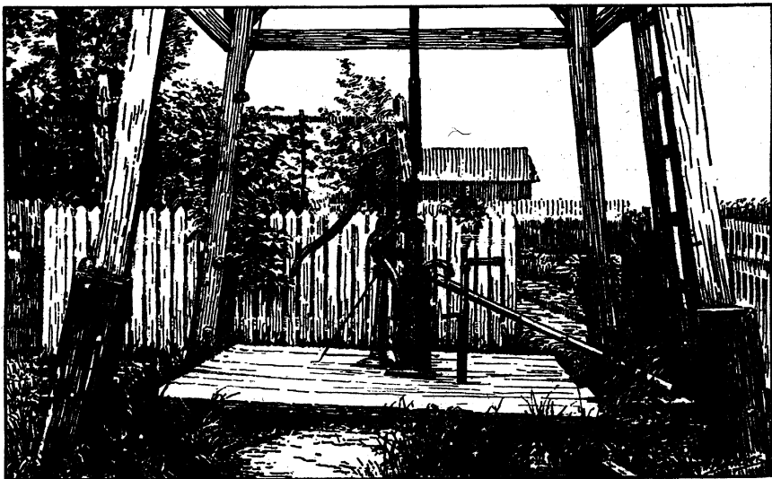
FIG. 39.—A well with surroundings protecting it from pollution.
