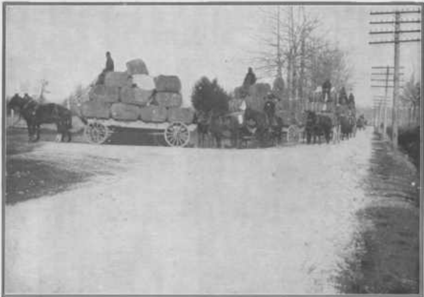
FIG. 2.—JUNCTION OF CHESTER LEVEE AND BEMIS ROADS, NEAR JACKSON, TENN. [This road was built of novaculite gravel, shipped from quarries in Illinois by Samuel Lancaster, city engineer, at a cost of $3,500 per mile.]
