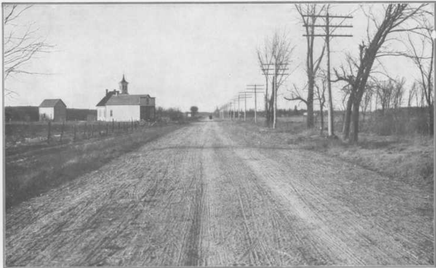
OSSEO MACADAM ROAD, 5 YEARS OLD, 3 MILES NORTH OF MINNEAPOLIS.
