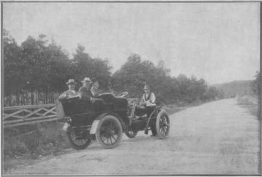
FIG. 1.—THE JOPLIN, MO. SPECIAL ROAD DISTRICT COMMITTEE INSPECTING THE FINE ROADS CONSTRUCTED OF MINING SLAG UNDER THEIR SUPERVISION. [There are about 100 miles of these roads, built at a cost of about $150,000.]
