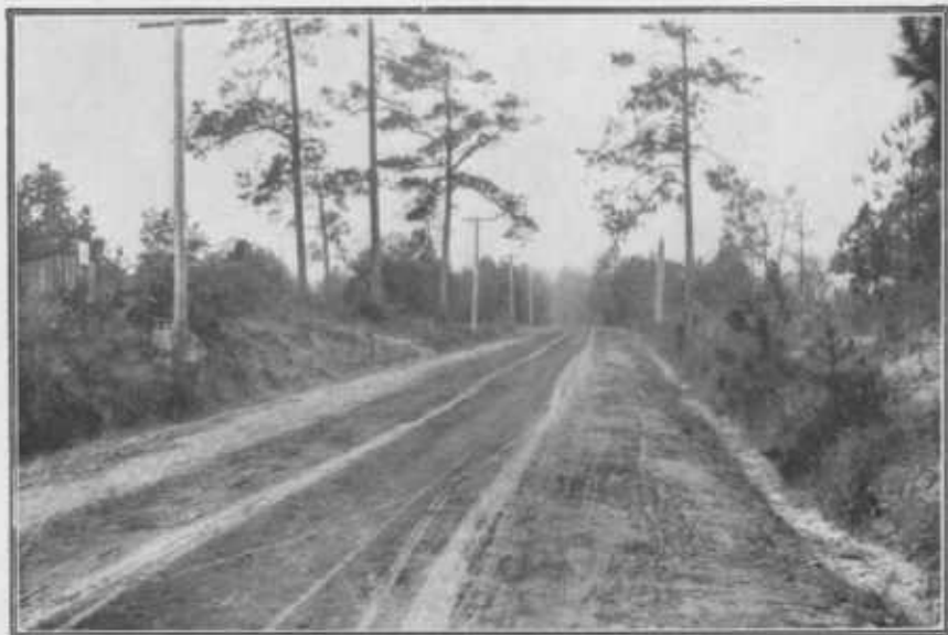
FIG. 1.—GARNERS FERRY ROAD, 3.5 MILES FROM COLUMBIA, S. C., USED FIVE YEARS WITHOUT REPAIRS.
