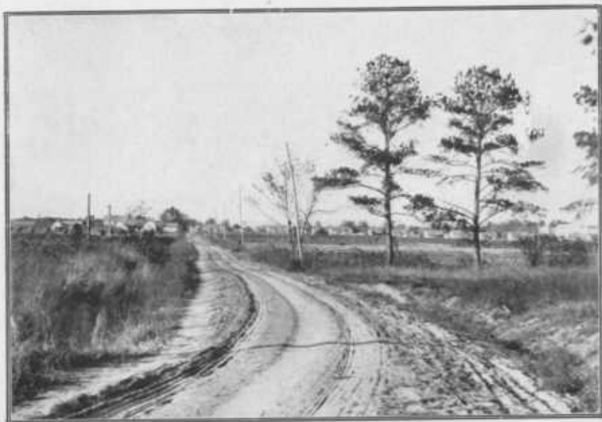
FIG. 1.—SAND-CLAY ROAD AT TARBORO, N. C. [Nothing has ever been done to this road since it was constructed.]
