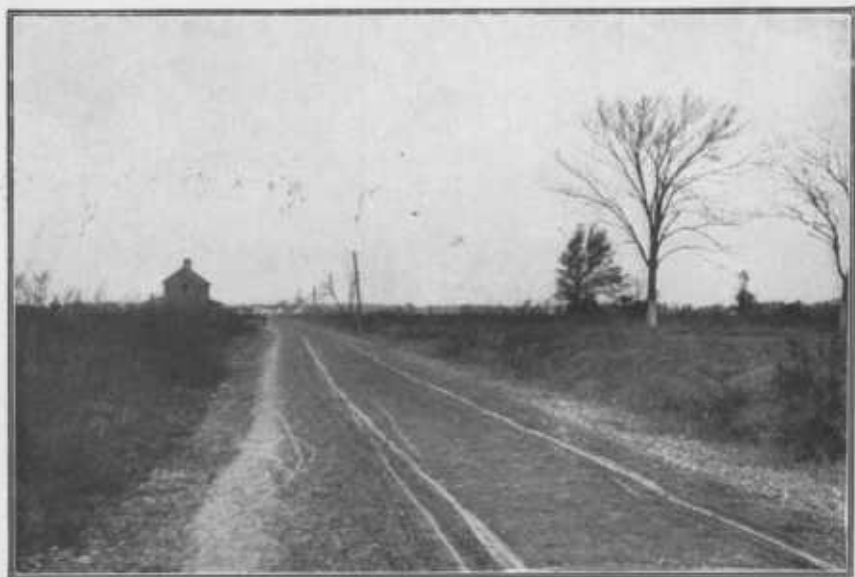
FIG. 2.—SAND-CLAY ROAD BUILT AT NEWBERN, N. C., UNDER THE DIRECTION OF THE OFFICE OF PUBLIC ROAD INQUIRIES.
