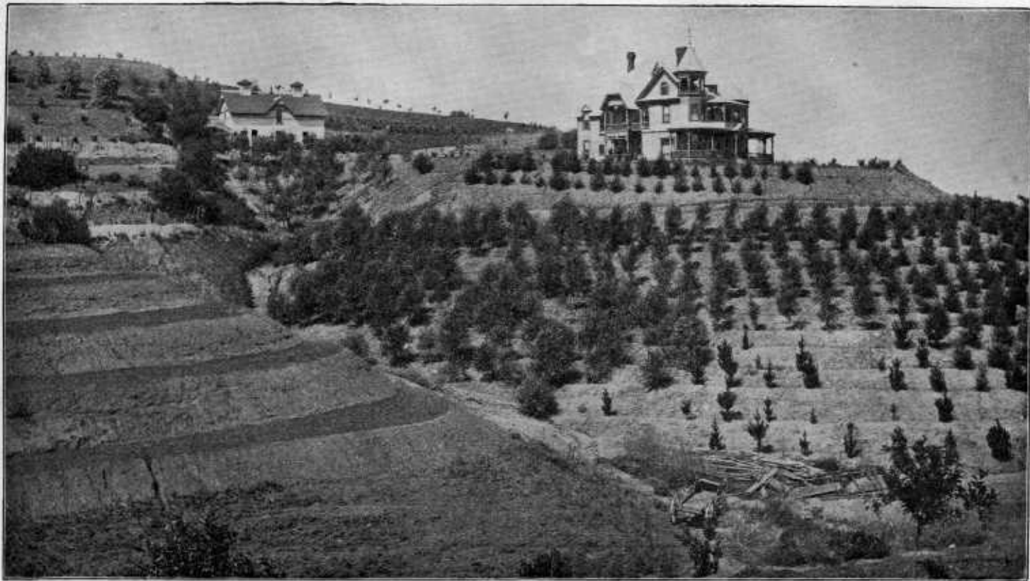
PLAN OF IRRIGATION BY TERRACES SHOWN AT THE LEFT OF THE RAVINE AND AN ORCHARD IRRIGATED BY CHECK LEVEES ON THE RIGHT OF IT.
