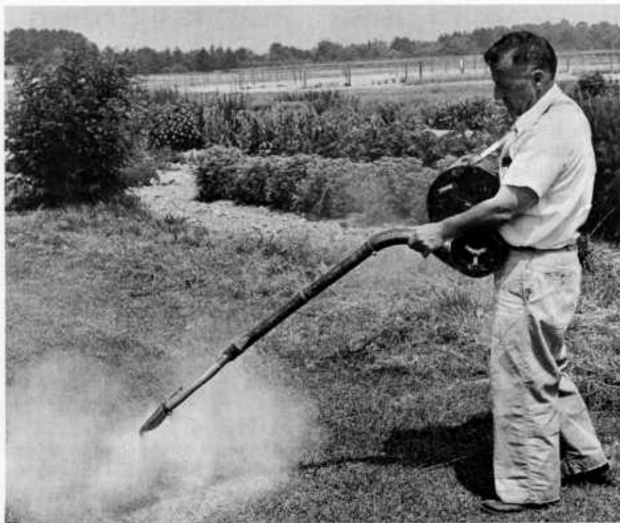
Applying insecticide with a rotary hand duster.
