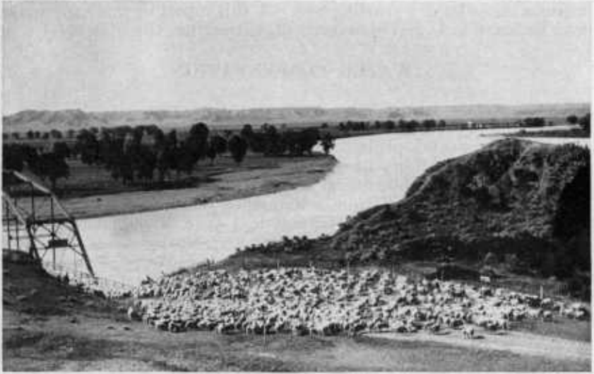
FIGURE 8.—Sheep crossing bridge, near Miles City, Mont.
