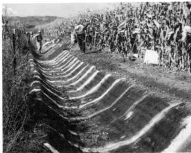
FIGURE 17.—Liner in place.
