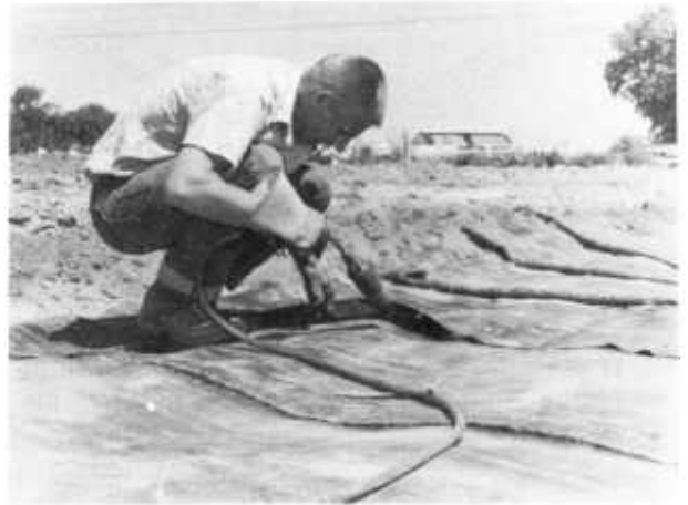
FIGURE 14.—Seaming widths of liner together with a torch.
