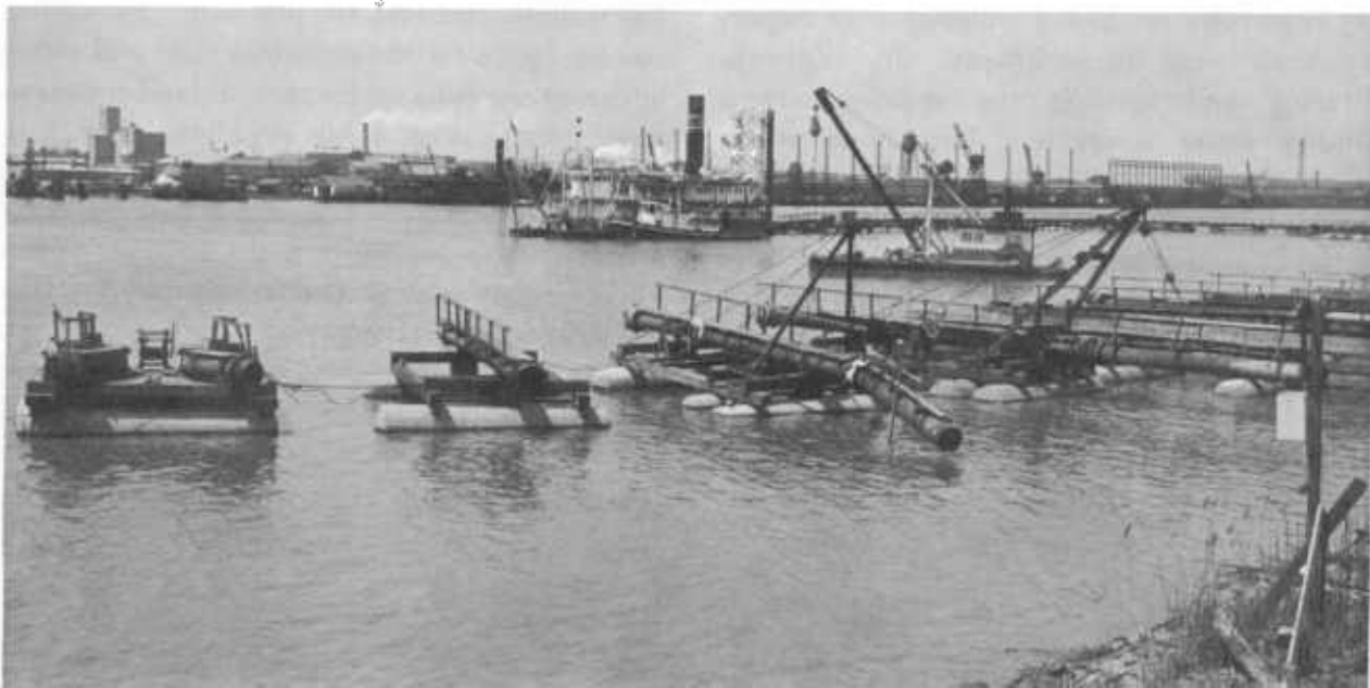
U. S. Corps of Engineers' dredge removing sediment—product of soil erosion—from the bottom of the Wilmington Harbor and Marine Terminal, Wilmington, Del.
