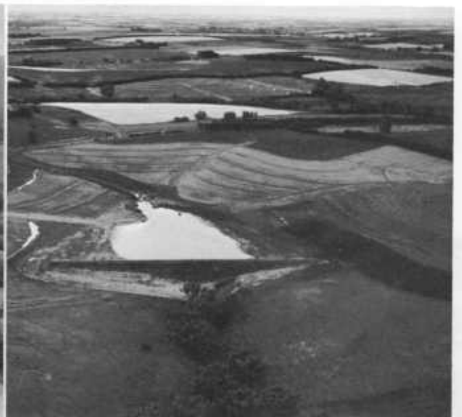
(Left) Willow plantings have stabilized this eroding streambank. (Right) Floodwater-retarding structures can help stabilize stream channels and keep gullies from spreading.
