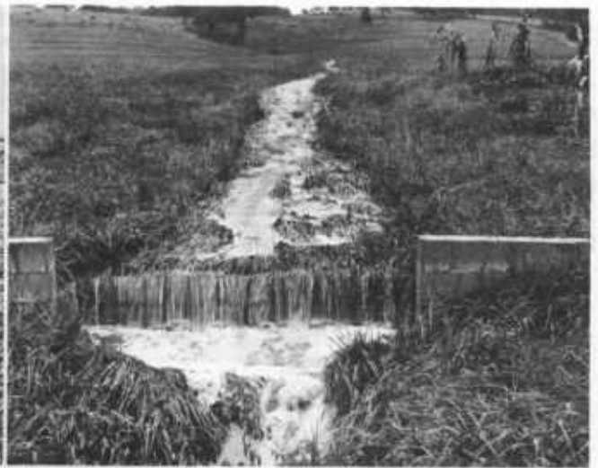
(Left) Terraces, such as these in Wisconsin, help reduce sheet erosion on cultivated land. (Right) The sod outlet and drop structure on this Indiana farm will help prevent gullies.
