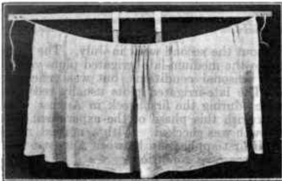
FIGURE 3.—Adjustable canvas check dam used in the head ditch to check the flow and to raise the water level
