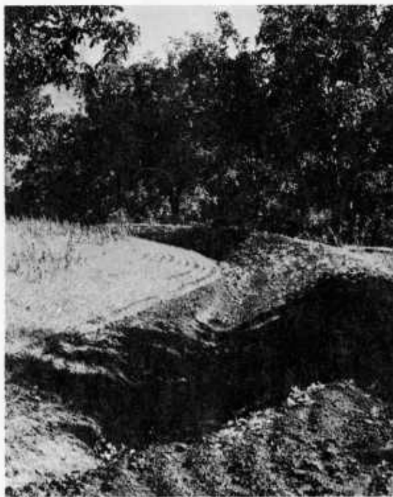
Terrace made of earth diverts water from upslope.
