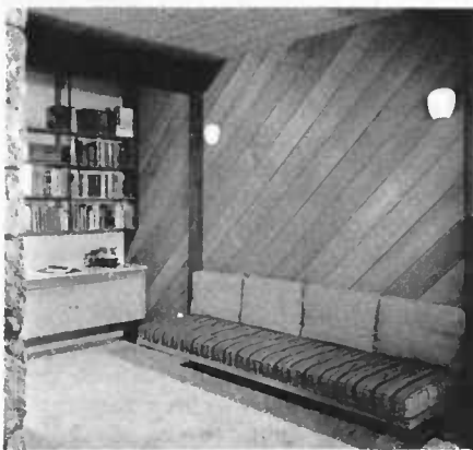
Top, rough-sawn, channel pattern western cedar wall paneling, repeated for cabinet front and doors. Family room formerly was basement storage area with unfinished concrete walls. Above, V-groove western red cedar boards applied diagonally on wall facing stone fireplace.
