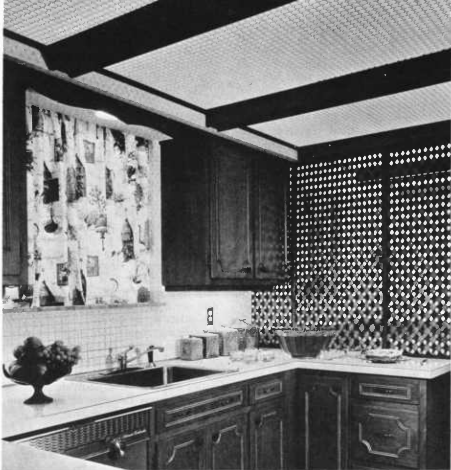
This kitchen features an entire ceiling of indirect light. Tubes are recessed slightly in the false beams so they can't be seen. Honeycomb material diffuses the light. Additional lighting is above the sink.
