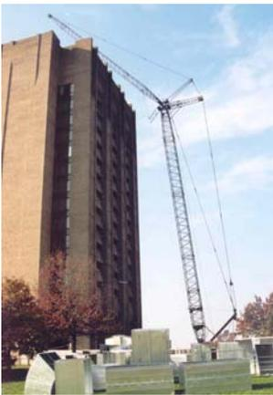
*The crane for the new air-handling unit #2 project lifts new duct parts to the roof of the NAL tower. (Click photo to enlarge.)*
