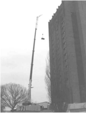
*Lifting part of the new air-handling unit to NAL's roof. (Click photo to enlarge.)*
