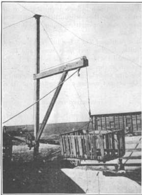
FIG. 3.—A simple type of hand hoist used in connection with a pit silo.
