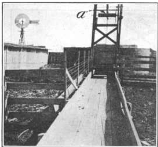
FIG. 5.—Another view of the silo and hoisting apparatus shown in figure 4. This illustrates the continuous feed trough, the top edges being used as a track for the truck. The barrel of the windlass on which the hoisting rope is wound is shown at "A."
