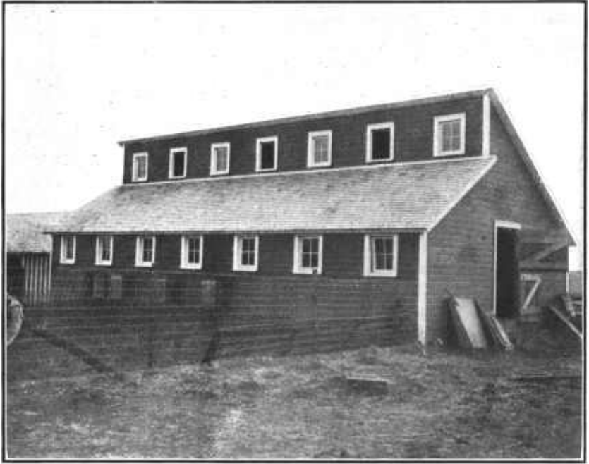
FIG. 3.—A substantial building, but with upper windows too high for locality where built unless late farrowing is desired.
