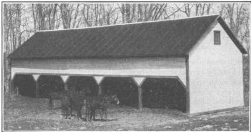
FIG. 10.—A shed open on the south side. A desirable place in which to winter colts unless the climate is too severe.
