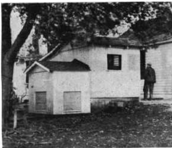
FIGURE 2.—A small shed with latticework sides built next to the milk room to house the compressing unit.
